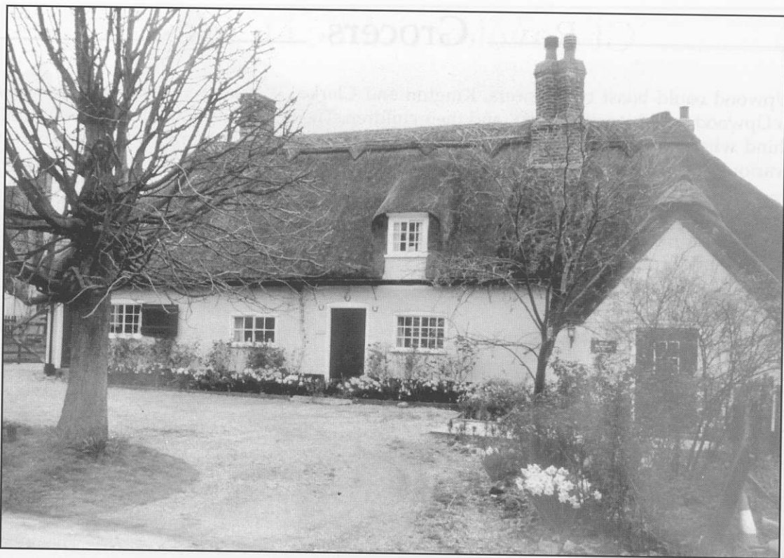
The Three Horseshoes public house, Gt. Raveley. This was, over the years, home to the local butcher and wheelwright.
